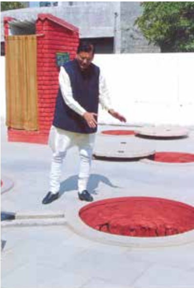
Pathak explaining how his two-pit pour-flush compost toilet works.
